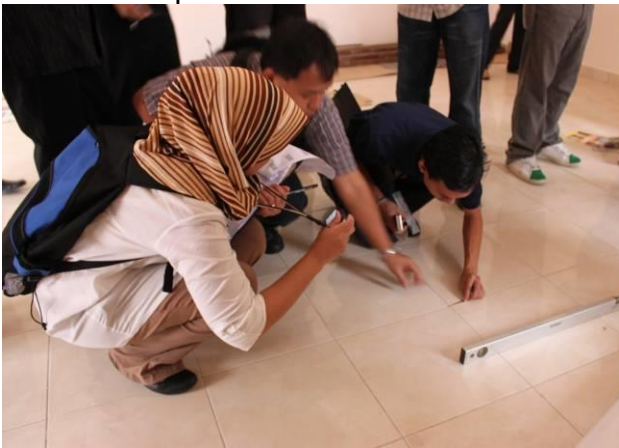
Trainees learning how to take measurement and recording of defects with inspection tools
