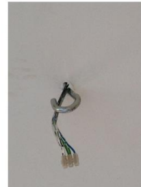
Proper fan hook connect to slab
