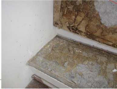
Termite attack at staircase
